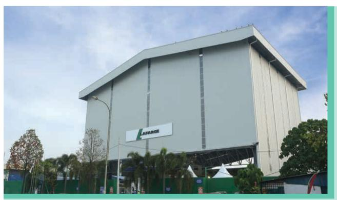
The Chan Sow Lin plant is Malaysia's first enclosed ready-mix concrete batching facility that is built to reduce noise and dust emissions and is capable of reclaiming returned concrete.
